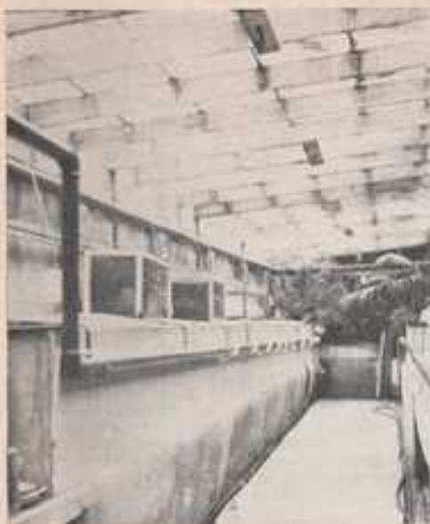
A view of a service passage between two rows of concrete tanks at Chester Zoo Aquarium, showing the overhead glass panels providing daylight illumination for aquaria.
