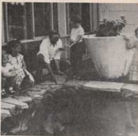
With the polythene pool filled with water, the edges of the plastic sheeting were anchored beneath stone slabs
