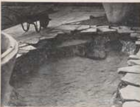
The excavation with sand-layered base ready to receive the plastic sheeting
