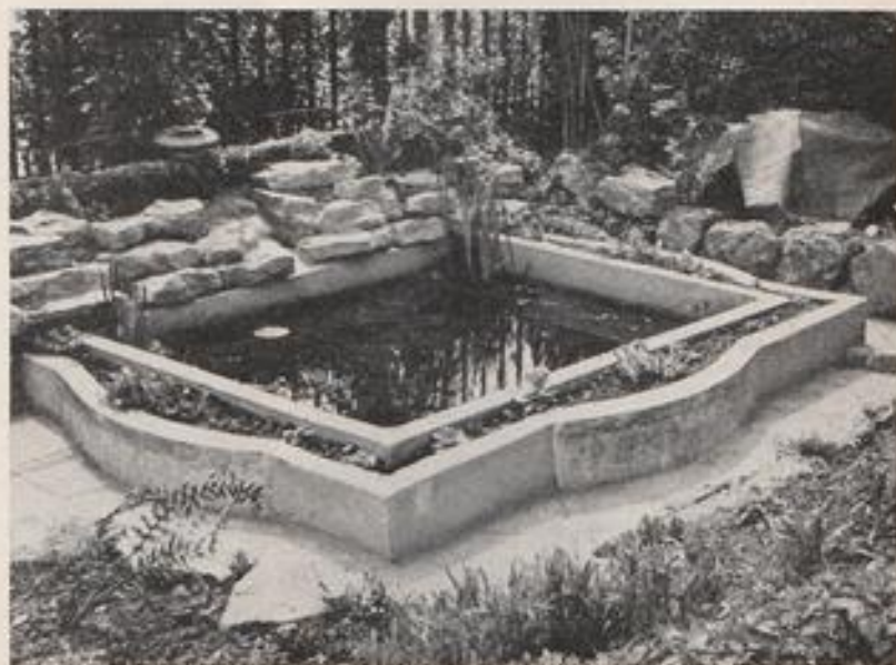
A pond made with a separate water-containing channel surround in which marginal plants can be grown in the loamy medium that these plants require
