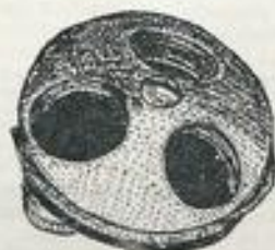
Modern triple nose-piece
