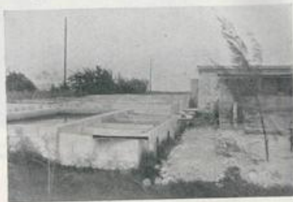
A view of some of the concrete tanks used for hatching and rearing at the Sumac Hatchery
