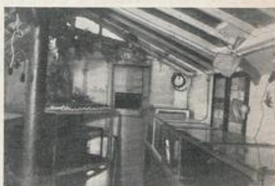
Another view of the house interior. The small doorway leads into the heating boiler annex
