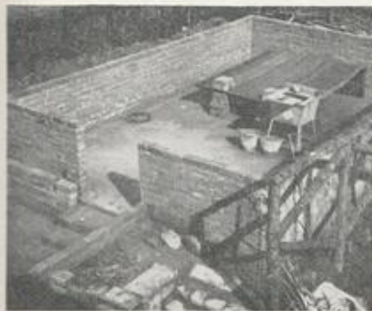
View of the completed outer brickwork of the author's fish house
