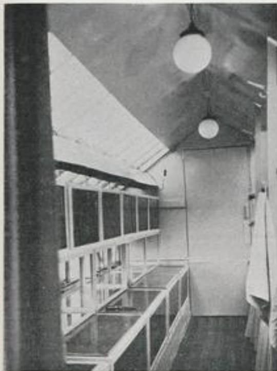
Breeding tank section of Mr. Foden's fish house. The glass panes in the roof are situated immediately over the aquaria, and good overhead electric lighting is also provided
