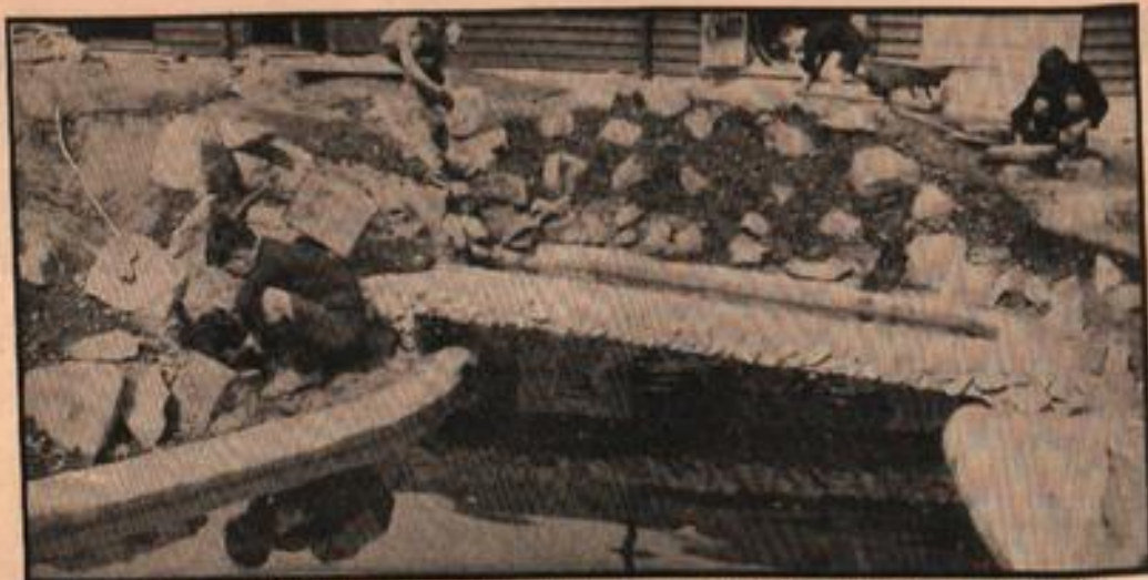
Fig. 5.—The pool filled, being tested for leakage. The boys are making a start with the surrounding rockery.
