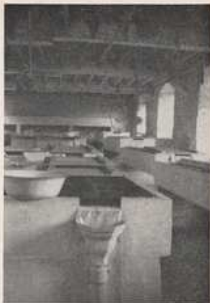
Step-down arrangement of large sinks in the Nailsworth trout-hatching house. Fresh water passes through the sinks continuously. In the sink nearest to the camera hatching trays can be seen.
