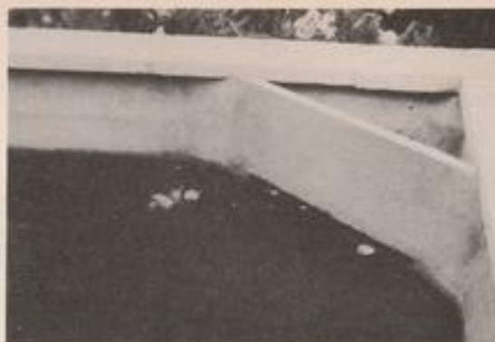
Above: The completed corner and water over-flowing slot about \frac{1}{2} " x 2".
