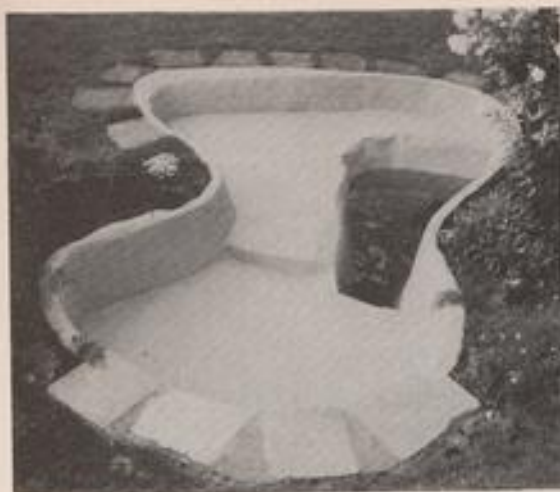
A concrete pond of varying depths ready for filling.
