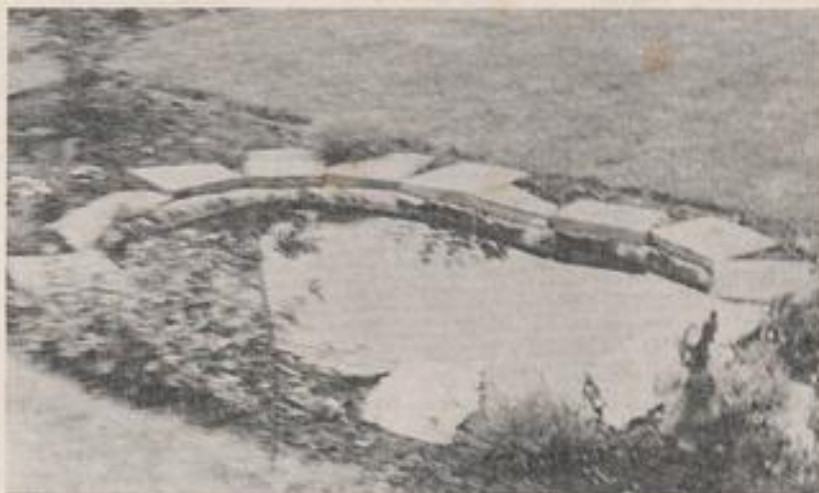
The writer's pond of plastic-sheet construction.
