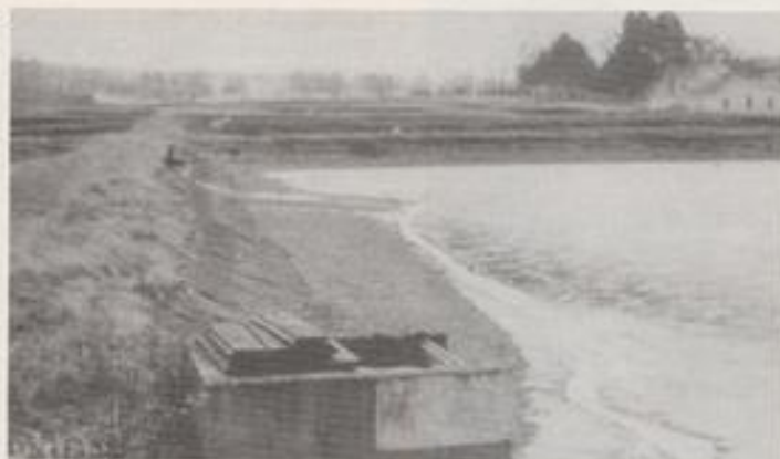
A typical breeding pond, shown here dried for the winter to kill off aquatic parasites, has its own intake pipe, its own discharge vent (operated by removing boards sequentially until the correct level is reached), and slopes covered with concrete to minimize siltation of the eggs
