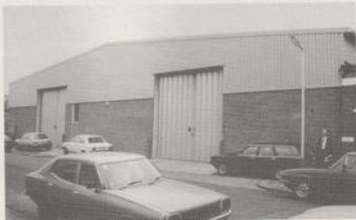
The new warehouse built on the site of the fire
