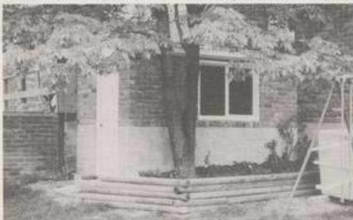
A Fish House built out of brick and concrete block and blending nicely with the house and deck area. This project gave a Fish House 7 ft. 8 inches wide and 11 ft. long. No problems were encountered with a service supply since water and electricity were just run in through the house wall
