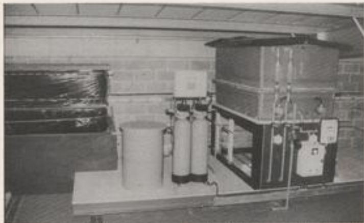
"Water hardness" cylinders are connected to fully automated header tanks where temperature and other final adjustments are carried out
