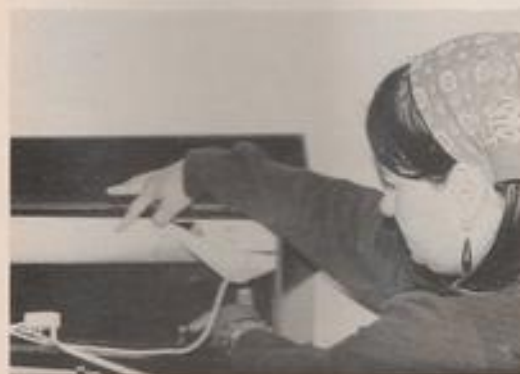
Barbara, the author's wife, points out the screws which do the main job of holding the unit to the wall. These are hidden by the coloured pvc sheet Barbara is holding out of the way with her right hand, when the tank is installed
