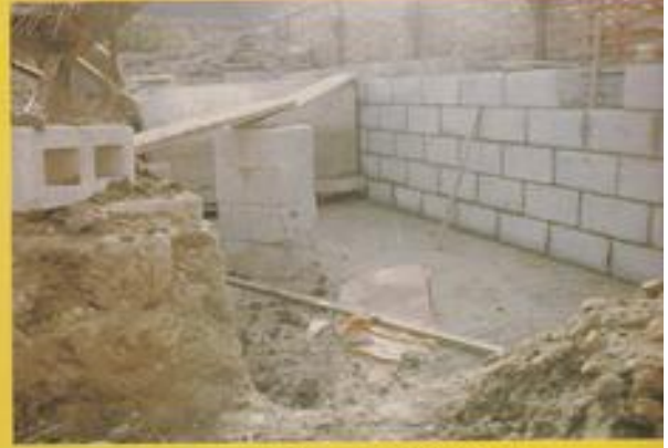
View of construction from within the pool
