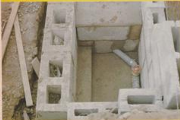
Pump house and main drain valve
