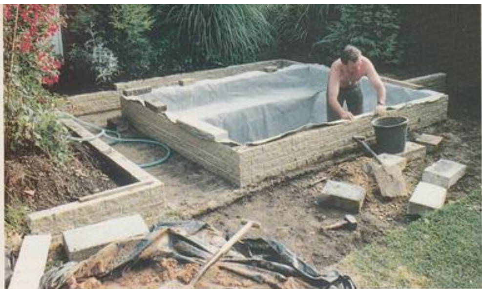
Blocks, cement and liner being incorporated into a formal raised set-up.
