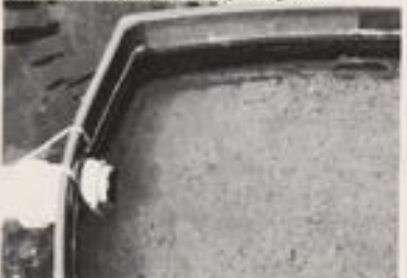
Left half, a box filter which has not been backflushed for a long time. Note the build-up of waste matter.
