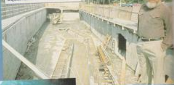
Kelly Tarlton back in 1983 by the foundations for the 'viewing tube' he planned for his new kind of public aquarium.
