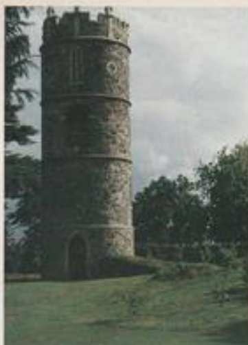
This tower at Goldney Hall in Clifton (Bristol) once supported an enormous beam engine or primitive steam engine that pumped water up from a well 300ft down to a fountain in a mock canal. Today's pumps are somewhat less obtrusive!
