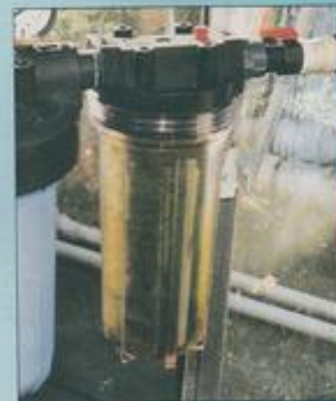
An example of what can happen if your purifier has a transparent prefilter housing fitted and it is kept in full sunlight. As you can see, the algal growth is considerable and has prematurely blocked the prefilter cartridge.
