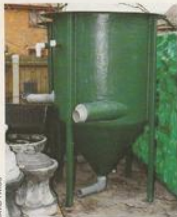
A modern free-standing (but usually located in a pit) vortex chamber. Such units are excellent for settling and disposing of solid wastes.
