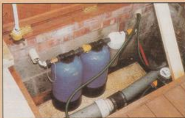
My MMR purifier "plumbed" into my pond system — all new water passes through it on the way to the pond.
