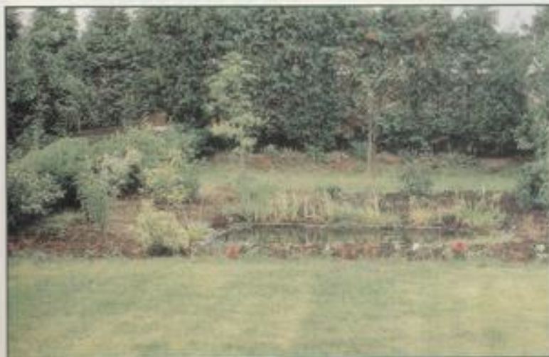
Shortly after completion and the rushes are already beginning to take over. The water level has been lowered to show the wall used to hold the earth back on the marsh area. PHOTO: D. CAMBERG
