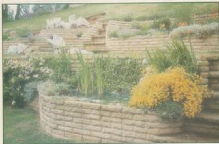
Almost finished! Pond built into wall using concrete.
