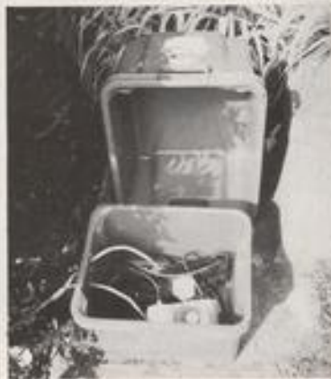
A tip for plugging pond equipment to the mains, or for housing transformers: use two sizes of plastic 'tidy' boxes (usually on offer at DIY stores); place the larger box upside down over the lower to give protection from weather and insects, etc. allowing domestic plugs and sockets to be used. This is protected by a mains circuit breaker, of course. If in doubt, consult a qualified electrician.
