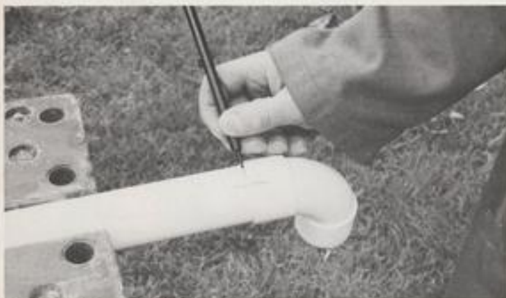
Mark depth of socket and rotational position.
