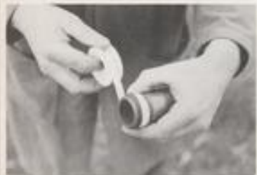
Applying P.T.F.E. tape to a male thread.
