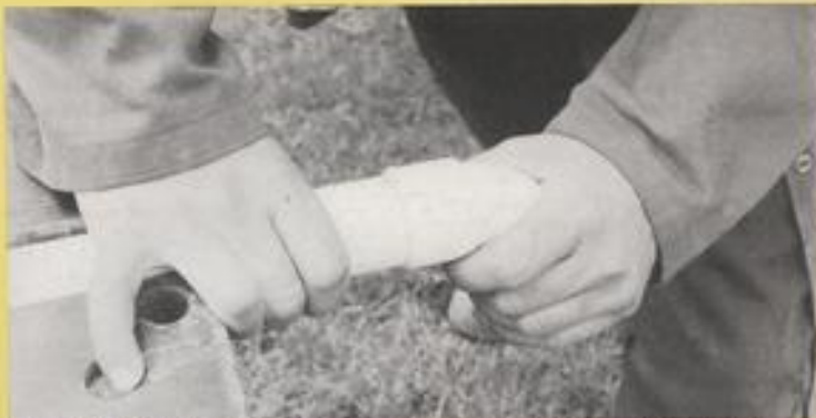
Push the pipe into the socket and adjust it immediately to correspond with the marks.
