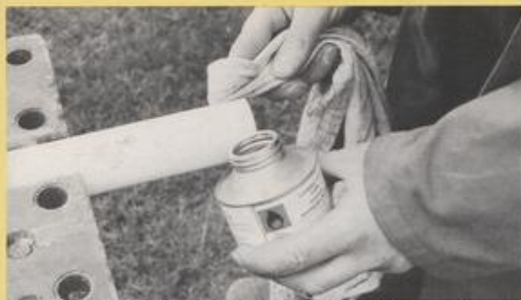
Alternatively, solvent cleaning fluid may be used for preparing the pipe and socket.
