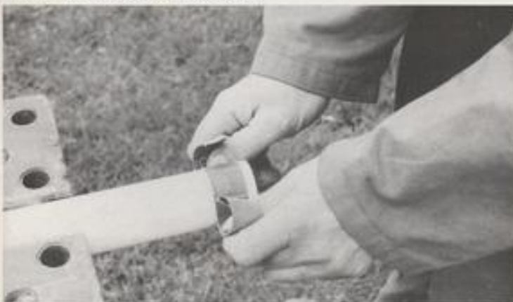
The pipe and socket can be prepared with abrasive paper.
