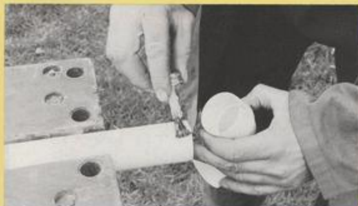
Apply solvent cement to pipe and socket.
