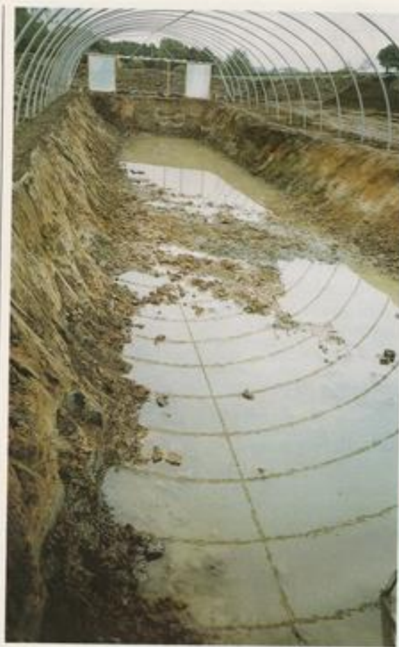
One of Treecircle's mud ponds under construction
