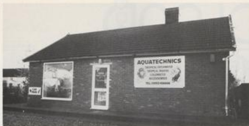
It may look like a bungalow... but this brand-new building marks the birthplace of one of the UK's newest aquatic ventures - Aquatechnics.
