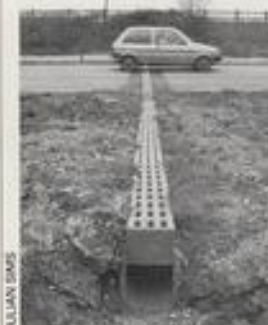
Ventilated ACO Toad Tunnel near Steyning. The low flexible polythene barrier is visible on the far side of the road.
