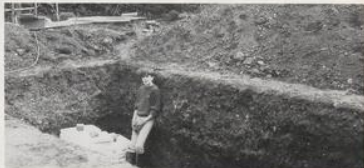
No. 2 son, Giles, shoring up the excavation during a lull in the day's digging. The temporary home for my then-existing collection of fish can be seen top left.
