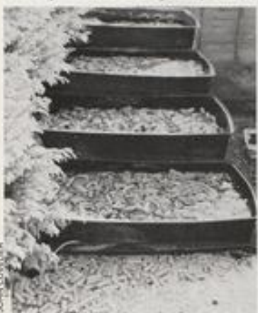
A DIY plumbers' tank filter. The staggered height achieves gravity flow from the pumped inlet via the pre-filter (seen at the far end).
