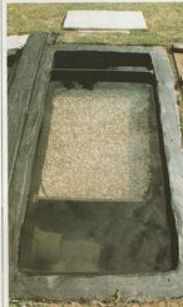
Completed biological filter prior to being put into operation.
