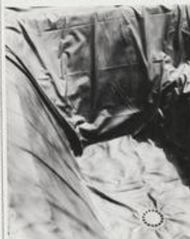
Butyl liner laid in position, with sealed and centred bottom drain.
