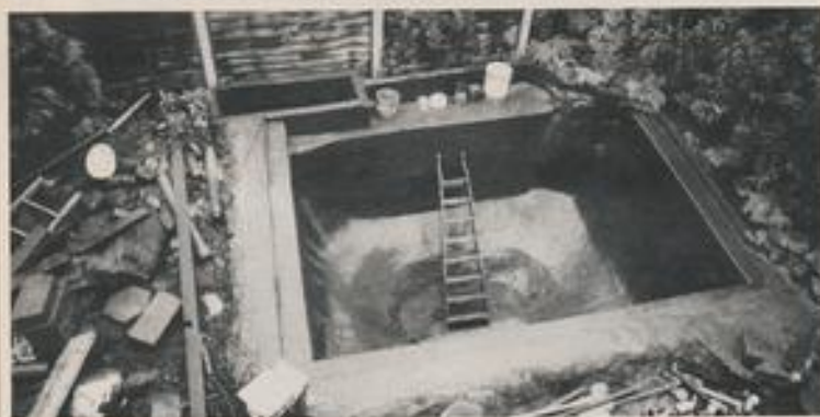
Stages in the construction of Mark 5.
