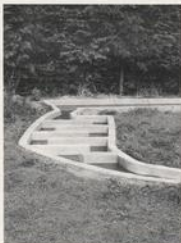
The rendering for the whole of this "partitioned" filter system contains Fibromix.
