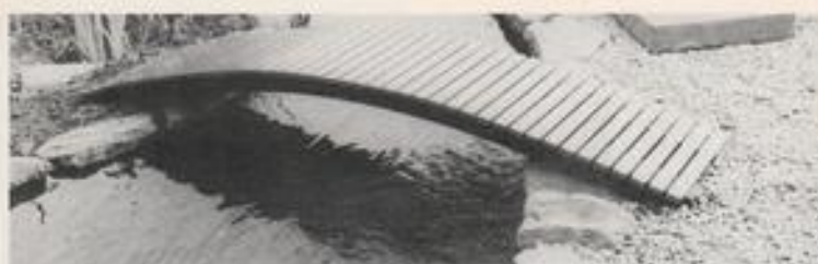
This simple bridge incorporates a cast concrete arch which had Fibromix added to the basic formula.
