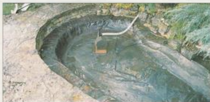
Lined pond with stonework built in from the marginal shelf upwards.
