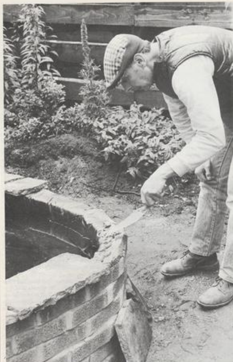
Adding the finishing touches to the pond.
