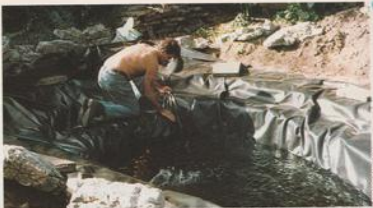
Plant and design your pond carefully. The correct size, depth, etc., must correspond to the types of fish you wish to keep. This pond, which will hold approximately 1500 gallons, is being constructed to hold a selection of Goldfish, Shubunkins, Golden Orfe and Tench.
